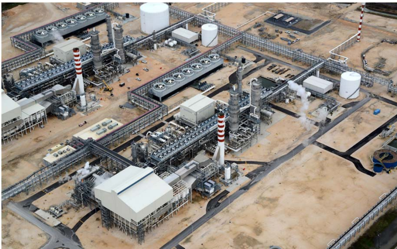
Completed Geismar 2 plant in operation*
