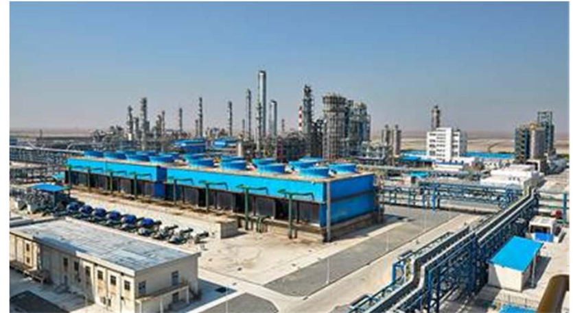
Ningbo Skyford's 1.8 MMT merchant methanol to 0.6 MMT olefins plant
