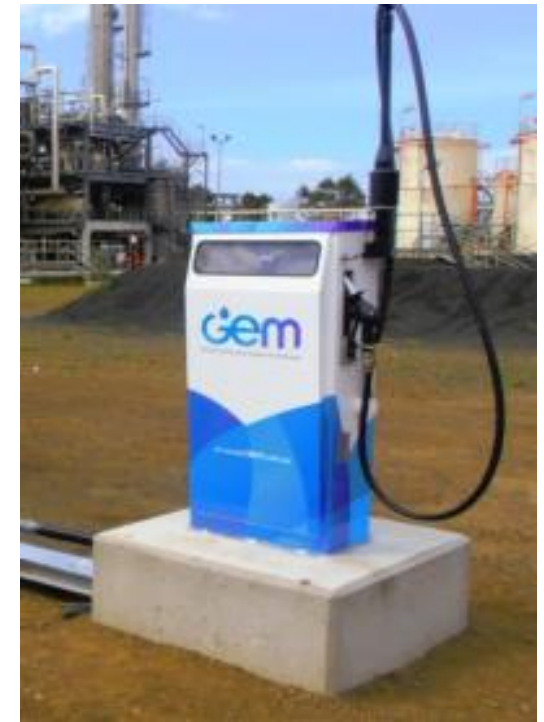
Methanol / gasoline pump at Coogee plant site
